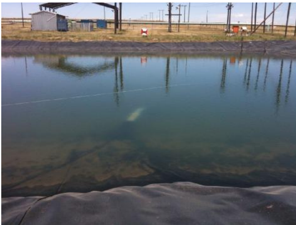
Figure B.2: Raised, lined earthen raw water dam
