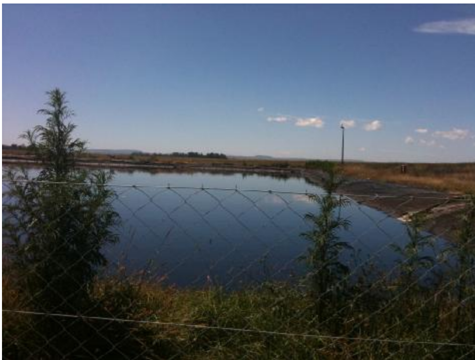
Figure B.1: Raised, lined earthen condense dam (for waste water from UCG process)
