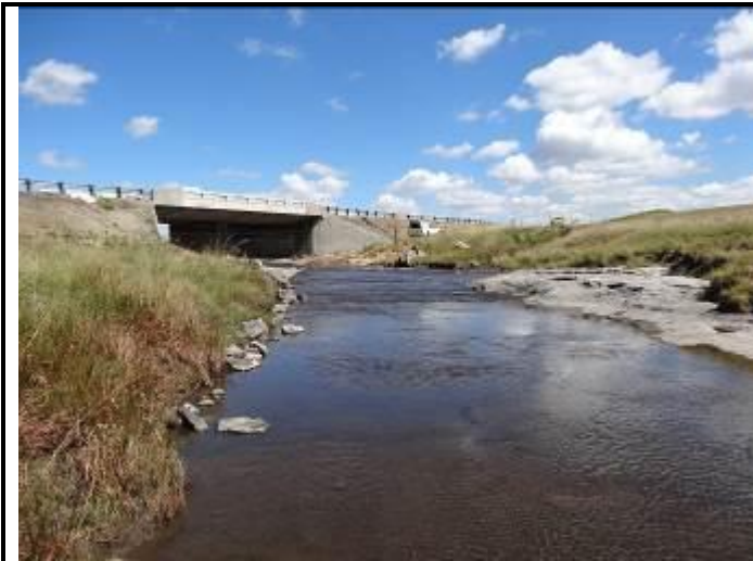
Figure 6: Upstream view of the GK2 site on the Geelklipspruit indicating the low flows at this point.
