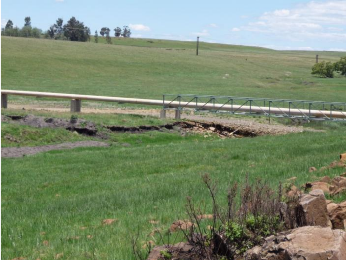
Figure 72 – Existing pipeline crossing the Witbankspruit near the demonstration plant
