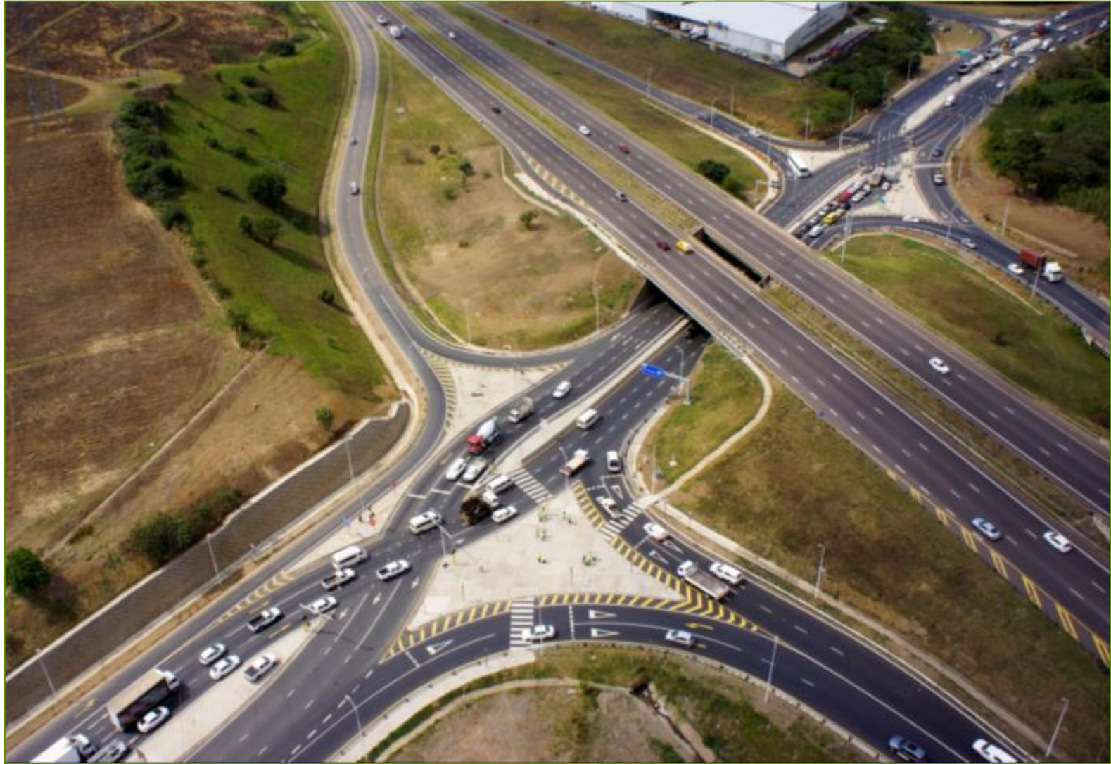
Figure 19: Diverging Diamond Interchange at N2 – KwaMashu designed by Aurecon South Africa (Pty) Ltd
