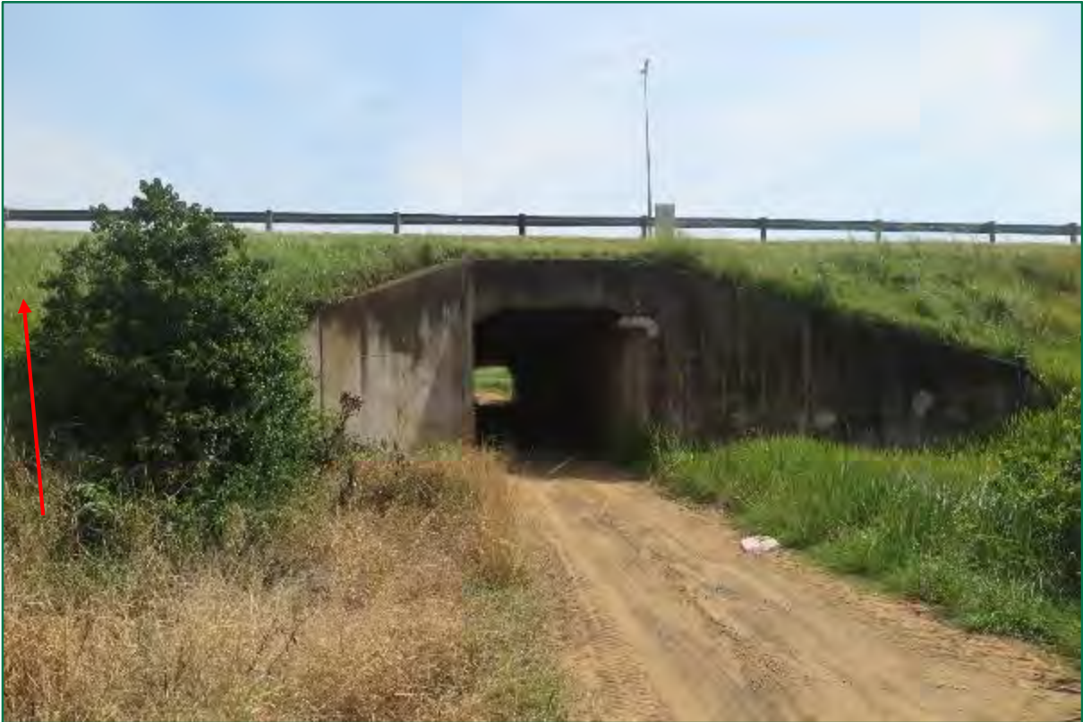
Plate 5: The red arrow indicates the pipeline alignment near the culvert that runs under the N2 on the eastern side. The vegetation considered to be scrubby and pioneer in nature.
