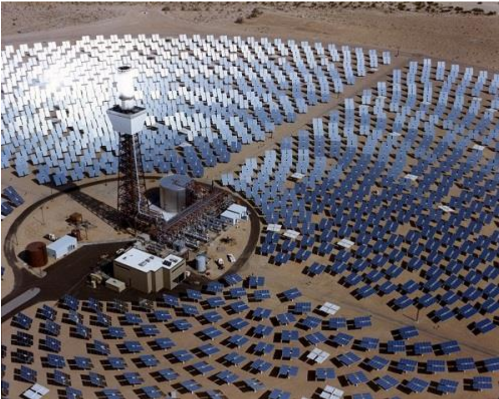
Figure 6: Example of central receiver.
