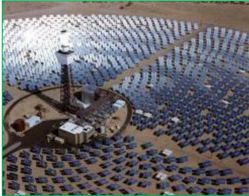
Figure 1-3: Example of a solar power tower system
