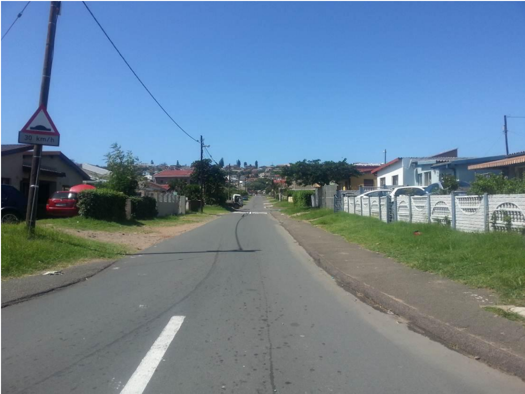
FIGURE 3-3 : FORMAL, DEVELOPED HOMES IN CLOSE PROXIMITY TO SWWTW
