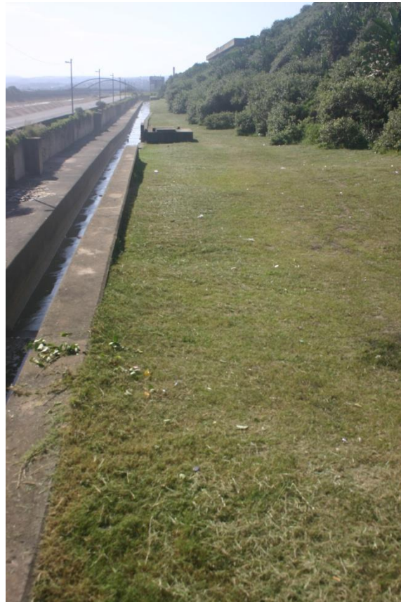
Plate 6: View of the mown strip of grass next to the Umlaas canal where the outfall pipe is buried on its way to the beach and sea (Fig. 3).
