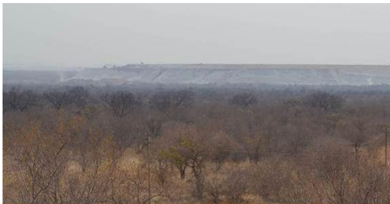
Figure 78: Southern face of the ADF as viewed from a high point to the south
