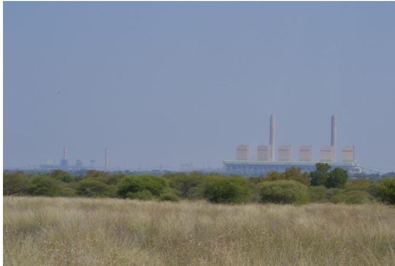
Figure 28: View of the Matimba (right) and Medupi (left) Power Stations from Lephale outskirts
