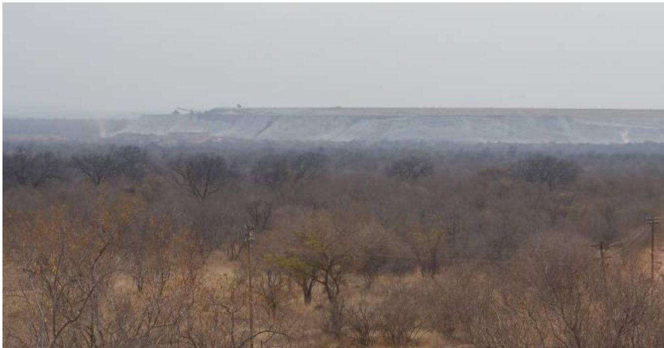
Figure 15 – The southern face of the ash dump as viewed from a high point to the south
