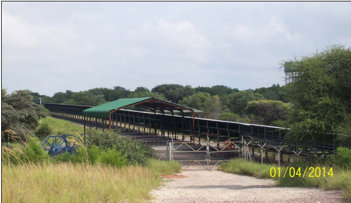
Figure 33: Example of a conveyor belt carrying coal from Grootegeluk Mine to Matimba Power Station
