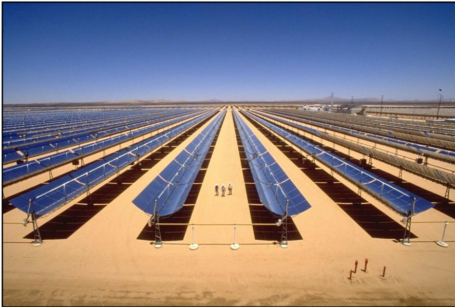
Figure 7: Parabolic field layout at the SEGS Plant
