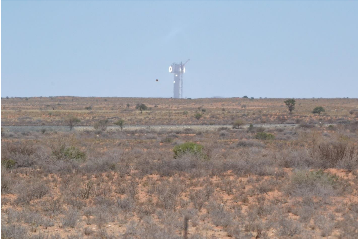
Figure 6 – An example of a central receiver CSP Plant as viewed from the N10 Highway near the Upington Airport
