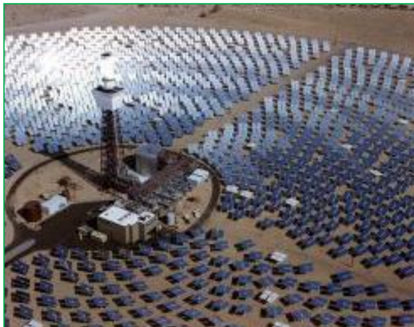
FIGURE 3: EXAMPLE OF A SOLAR POWER TOWER SYSTEM
