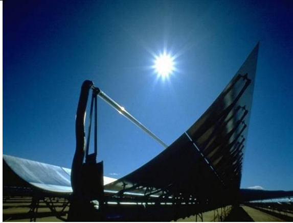
Figure 1: Photo of a trough system 1
