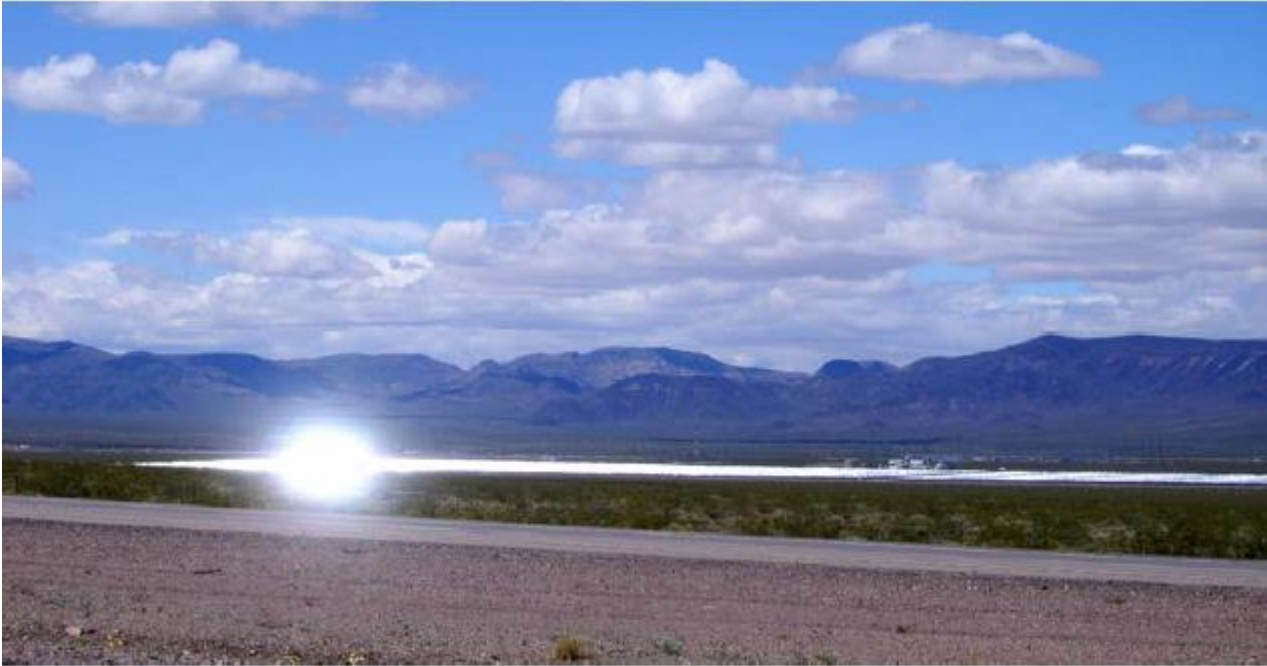
Figure 13 – Picture of a ‘glare spot’ at a parabolic trough facility in Nevada (Sullivan et al, 2012)
