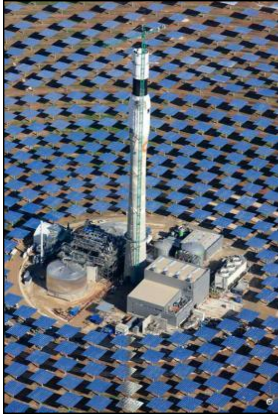
Gemasolar CSP Tower Plant with Molten Storage System
