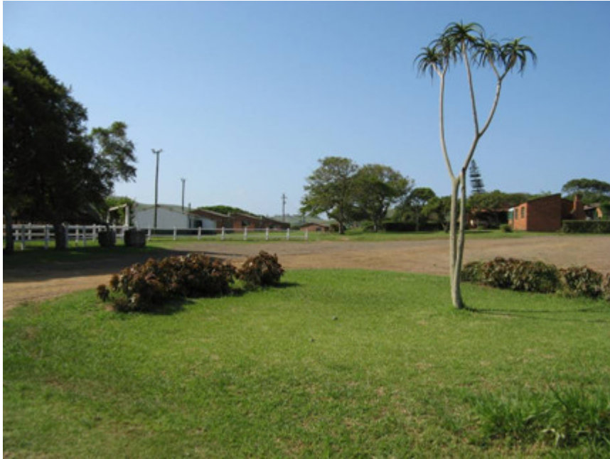
Photograph 9 Part of Accommodation, Administration and Workshop area at Blackburn Estate
