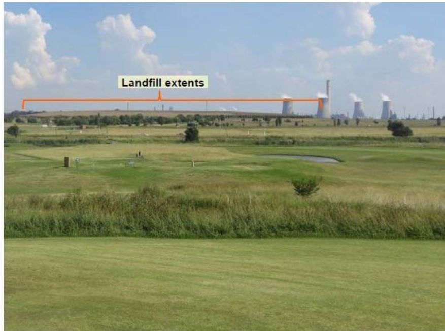
Tree screen and 15 m landfill height
