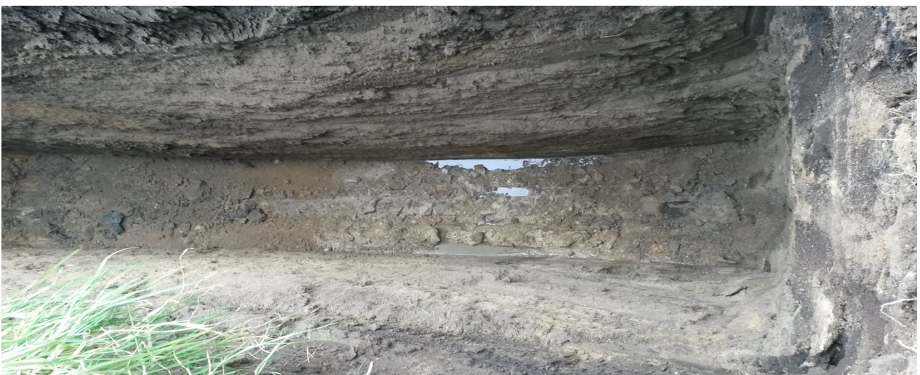
Figure 9: Seepage in Test Pit 1
