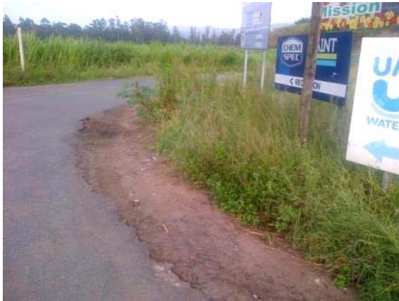
Photograph 6: Edge Failure
