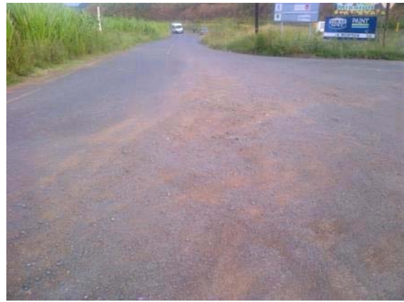
Photograph 7: Delamination
