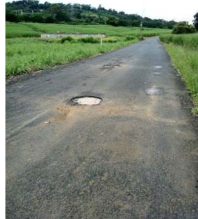
Photograph 4: P499 – Bad condition
