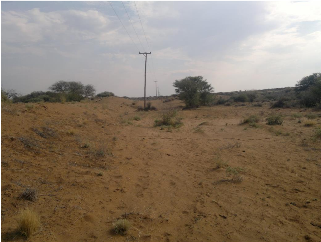
Figure 15 – Berm / impounding wall (left) constructed across the width of the watercourse at Crossing Alt1_13, with area behind in which water is trapped
