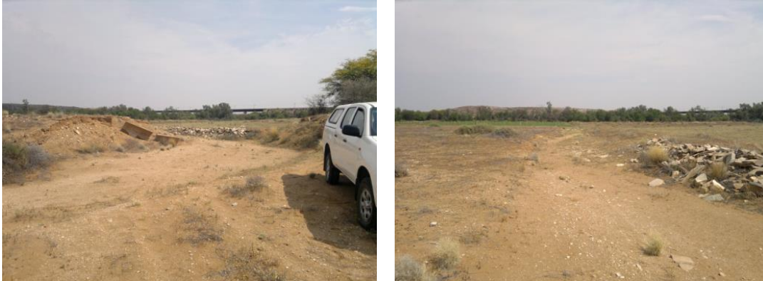
Figure 16 – Photographs indicating the degree of physical modification of the watercourse downstream of crossing Alt1_17 as it drains through the berm (left) and through the alluvial terrace (right)
