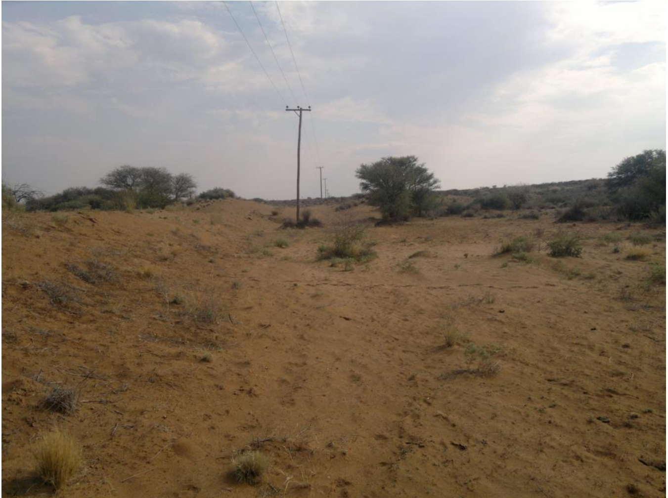
Figure 16 – Berm / impounding wall (left) constructed across the width of the watercourse at Crossing Alt1_13, with area behind in which water is trapped
