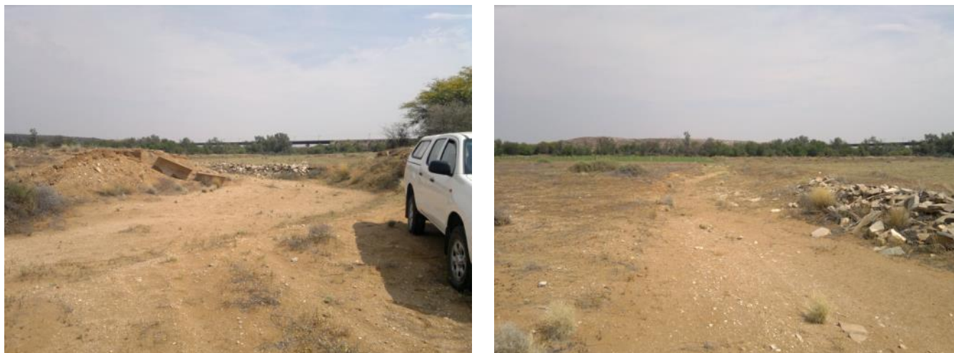
Figure 17 – Photographs indicating the degree of physical modification of the watercourse downstream of crossing Alt1_17 as it drains through the berm (left) and through the alluvial terrace (right)
