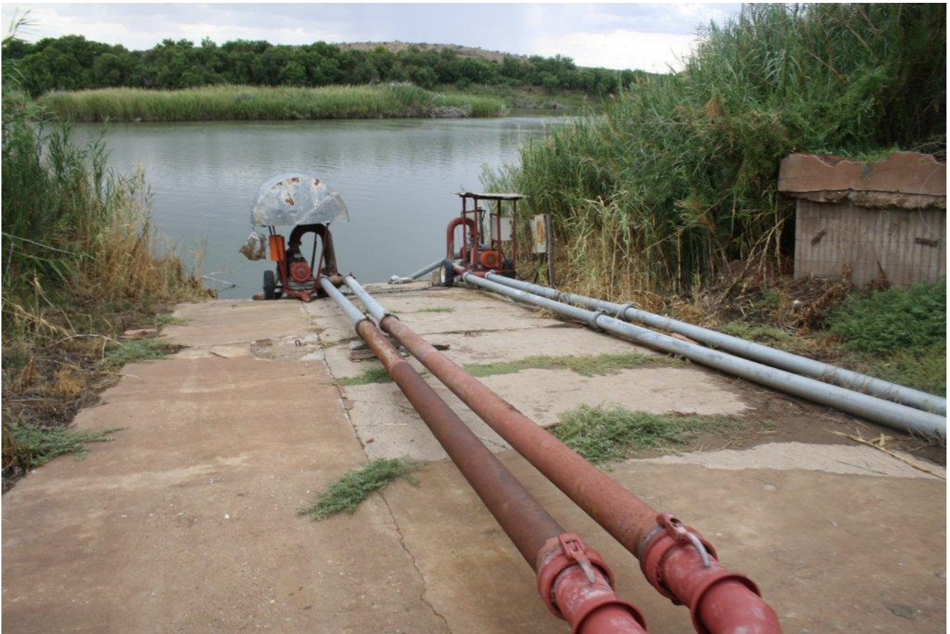
Plate 8: Alternatives 1 & 2 (West-facing) – The proposed new abstraction point (Shalom Point). Note: Existing infrastructure.
