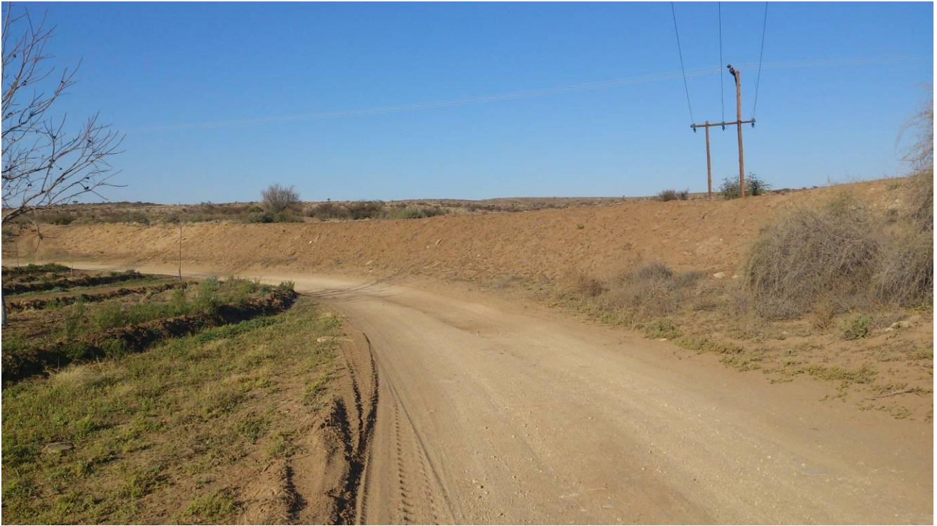
Plate 5: Alternatives 1 & 2 (East-facing) – The alternatives 1 and 2 meet at this point and the alignments are the same down to the proposed new abstraction point (Shalom point).
