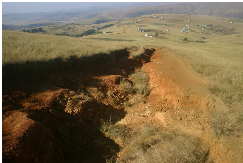
Plate 1: Erosion donga along an old gravel track from waypoint 42 to 48 in option 1 (Fig. 5).
