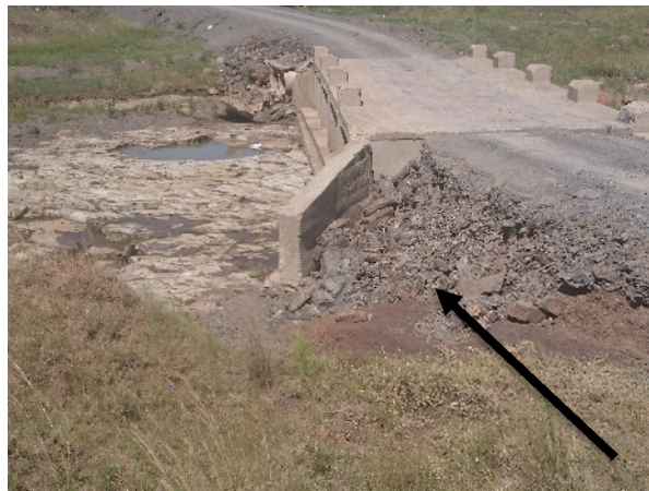
Photo 11: Example of erosion from road run-off entering a water course.
